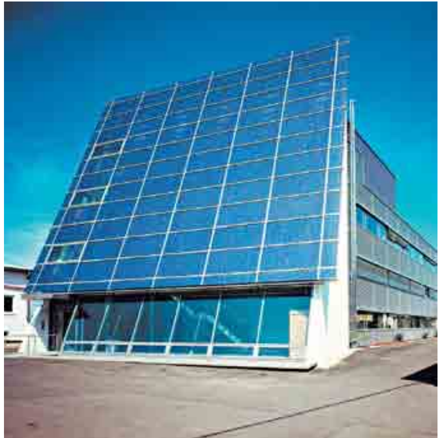
© SMA SOLAR TECHNOLOGY
